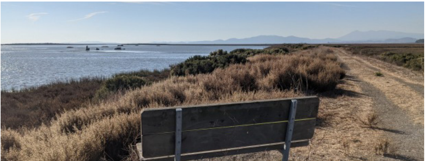
Top photo: Construction of a raised conventional levee in Foster City, CA, that was completed in 2024. Photo by the Foster City levee project. Bottom photo: Sonoma Creek Baylands restoration includes a nature-based adaptation in which the wetlands provide flood reduction benefits in front of a sloped levee. Photo by BAHiker.
