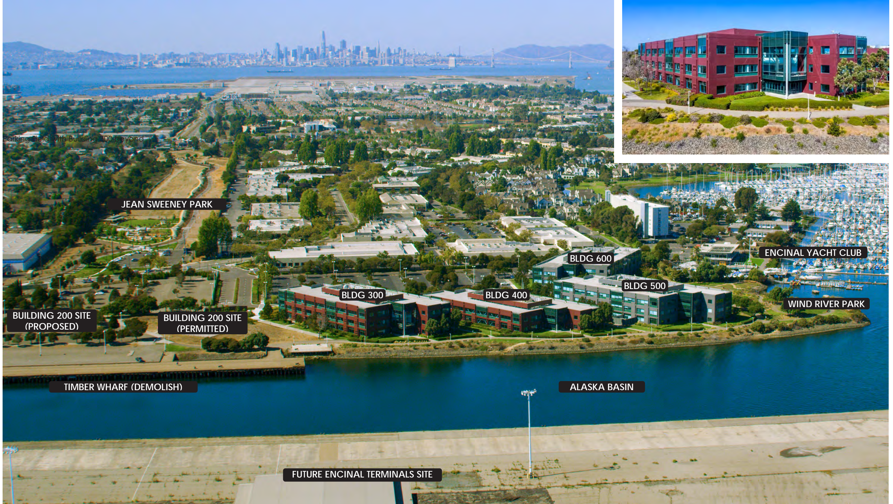
Existing conditions looking west towards Alameda Point. (INSET): Detail of Building 300 architectural character (400, 500, 600 similar)
