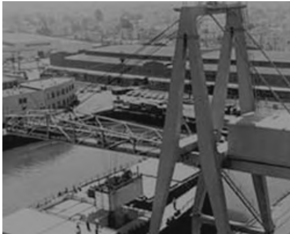
Crane used for unloading ships, sitting atop the existing timber portion of the wharf. Del Monte warehouse (now Alta Star Harbor housing) in the background, with Encinal Terminals on the left.
