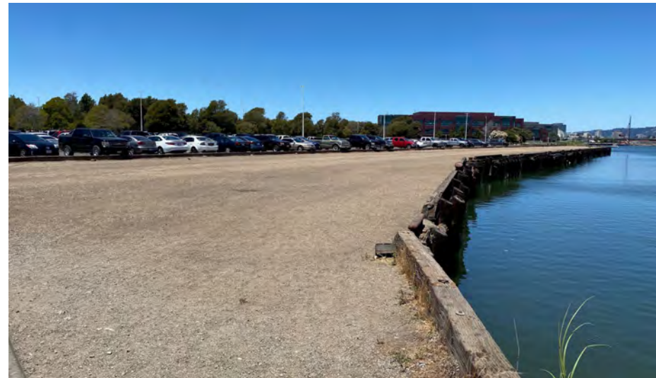
6. Edge of Timber Wharf Looking North Along Shoreline
