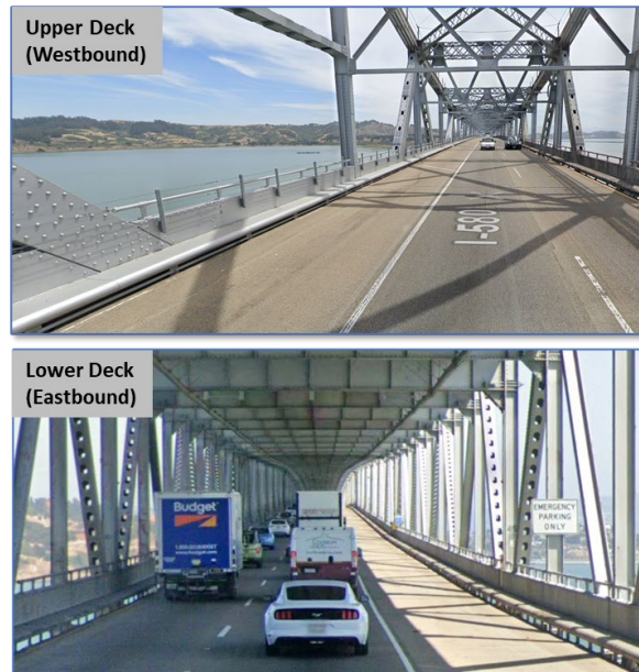
Figure 2-5: Initial Conditions – Bridge Upper and Lower Decks
