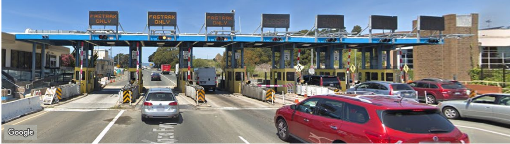
Figure 2-7: Approach to Richmond-Toll Plaza before March 2020
