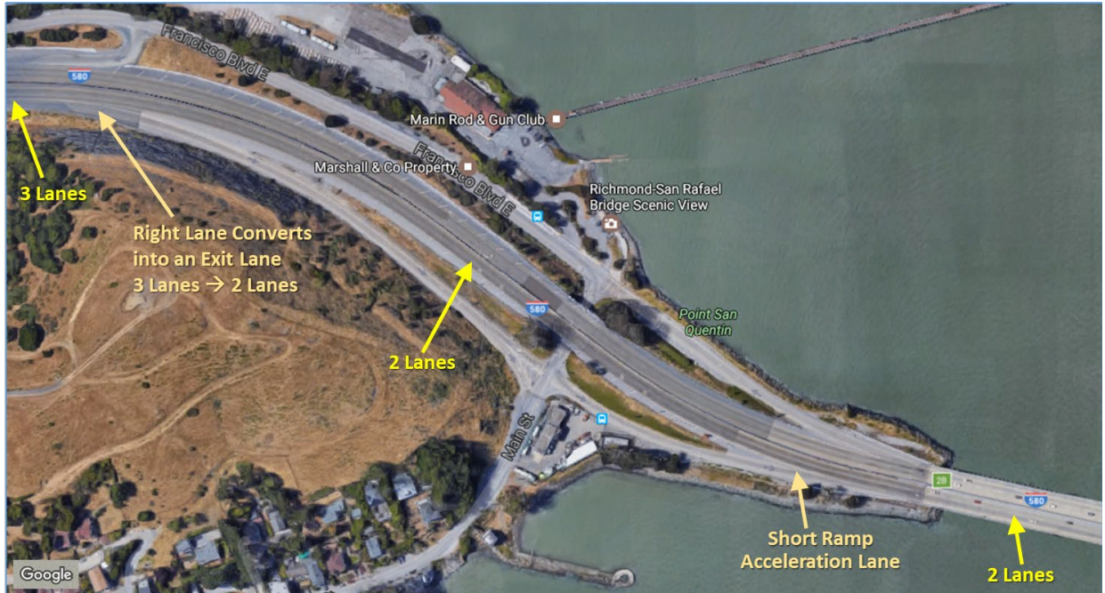
Figure 2-4: Initial Conditions – Eastbound Bridge Approach in Marin County
