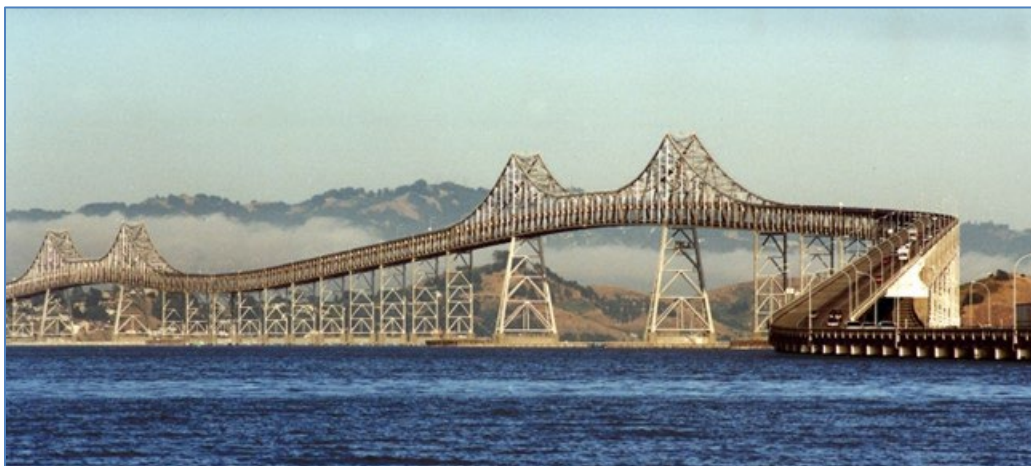
Figure 2-2: Richmond-San Rafael Bridge
