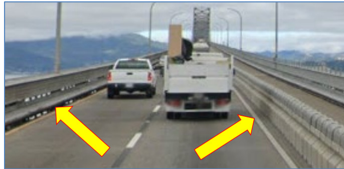
Figure 8-79: Relative Closeness Bridge Guardrail on the left and Path Barrier on the Right
