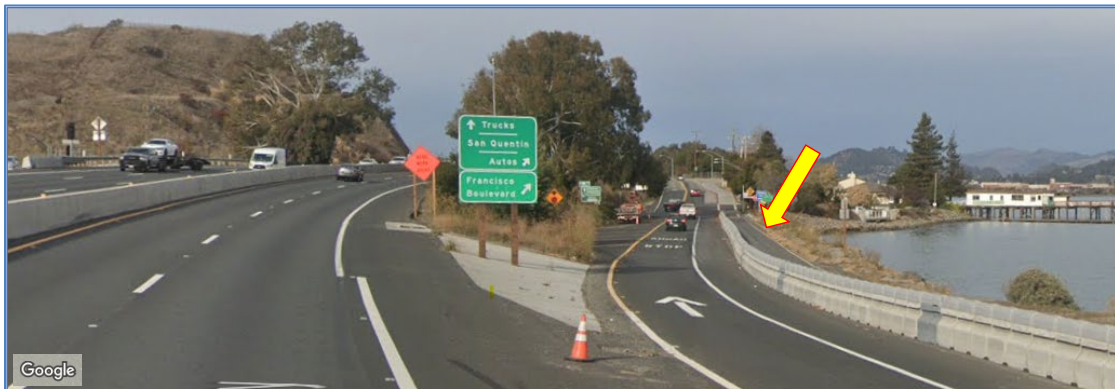
Figure 2-19: Bike/Pedestrian Path Western End Along Main Street Off-Ramp
