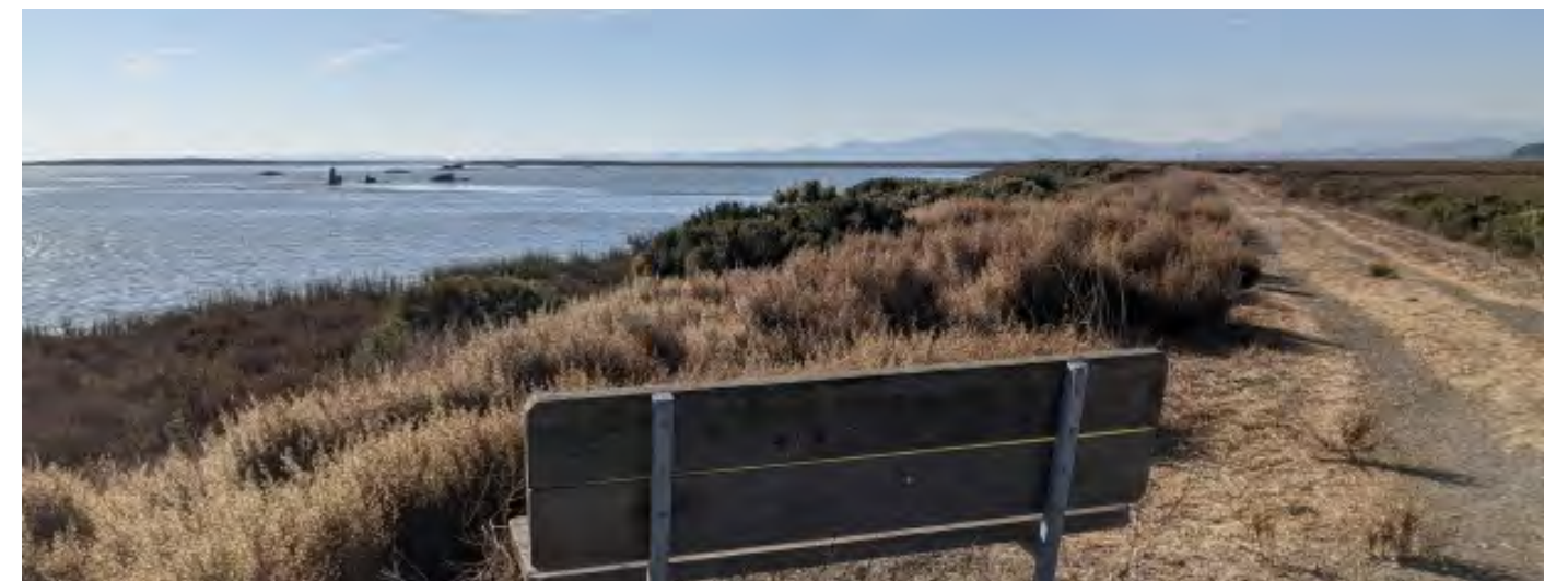
Top photo: Construction of raised conventional levee in Foster City, CA which was completed in 2024. Photo by the Foster City levee project. Bottom photo: Sonoma Creek Baylands restoration includes nature-based adaptation where the wetlands provide flood reduction benefits in front of a sloped levee. Photo by BAHiker.
