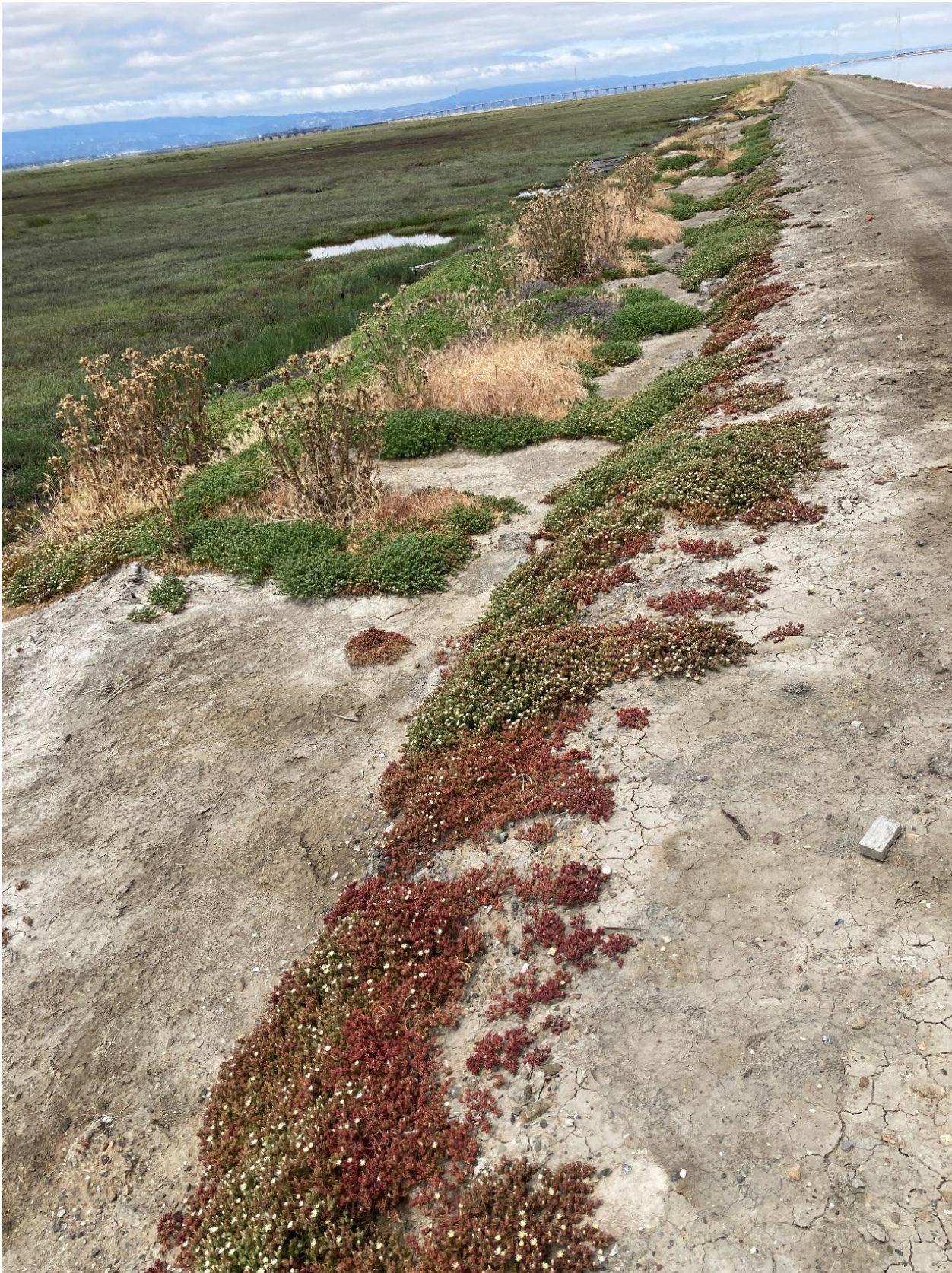
Photo 9. The outboard berm at Pond P2-12 showing the extensive tidal wetlands.
