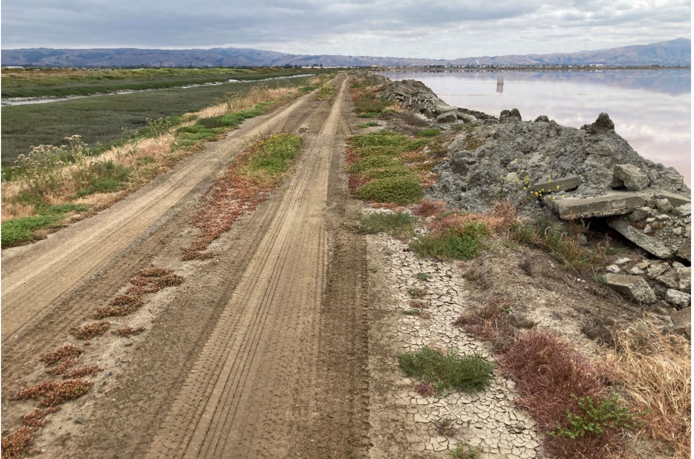
Photo 3. Looking east with the former barge canal on the left and Pond P2-13 on the right. This berm is drivable only during dry weather.
