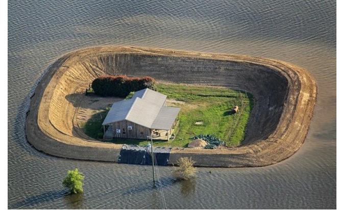
A levee protects a home surrounded by floodwater from the Yazoo River, near its confluence with the Mississippi River, on May 18, 2011 near Vicksburg, Mississippi. (Photo: Scott Olson) ( Mississippi Island Homes Are Just Class Apart | How Did They Do It ? | Reckon Talk )
