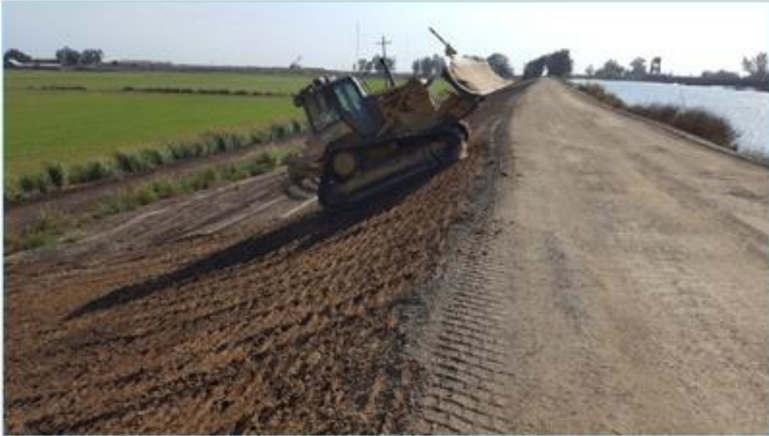
Maintenance being conducted on Delta levees.
