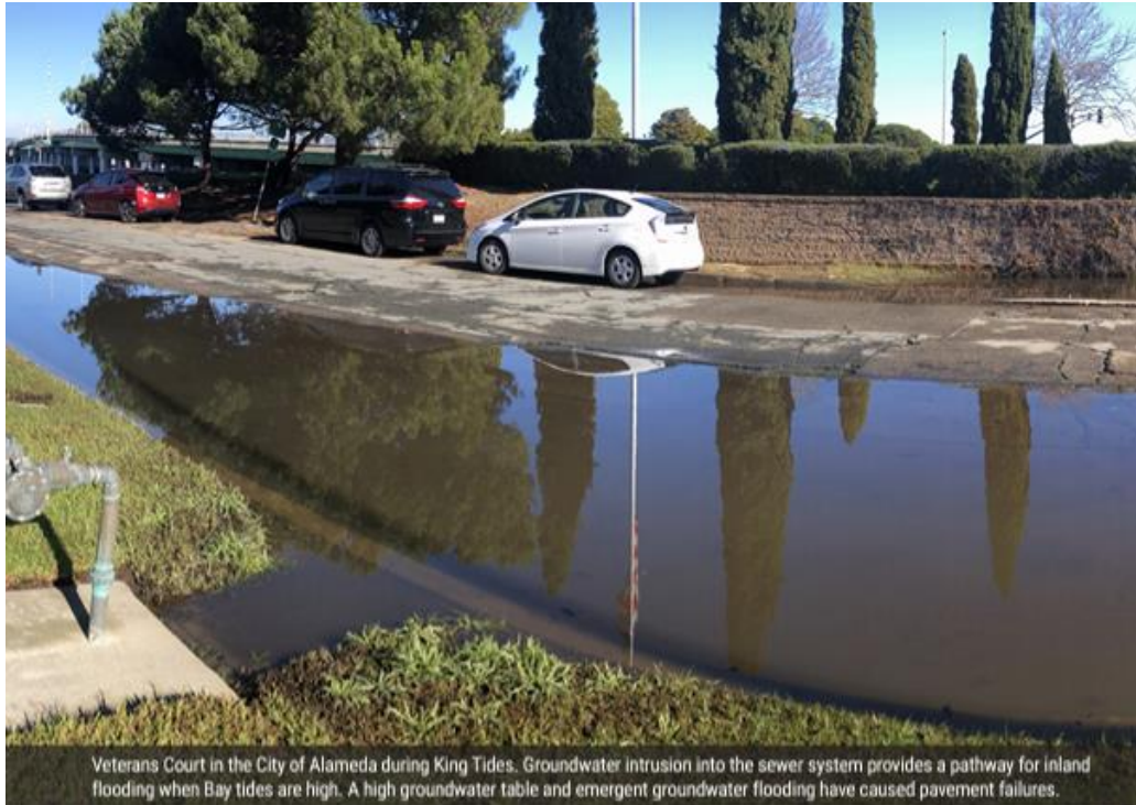
Photo of sunny day flooding from groundwater rise, from Shallow Groundwater Response to Sea-Level Rise by Pathways Climate Institute and SFEI, 2022.
