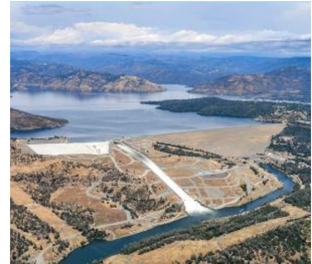
Oroville Dam and Spillway from https://water.ca.gov/News/Blog/2023/June-23/Oroville-Update-6-16-2023
