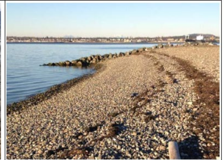
b) Boulevard Park, Bellingham; single larger groin at down-drift end of 280-ft-long beach.
