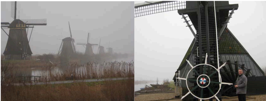
Figure 7. Many windmills built in the 18 th century have been preserved, such as this impressive line of mills at Kinderdijk, which is a UNESCO World Heritage Site. Technology of such windmills is intriguing; the whole top can be turned following the wind direction.
