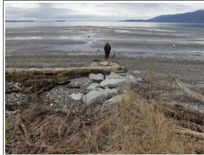
a) North Beach, Samish Island; single drift sill at down-drift end of 850-ft-long project.
