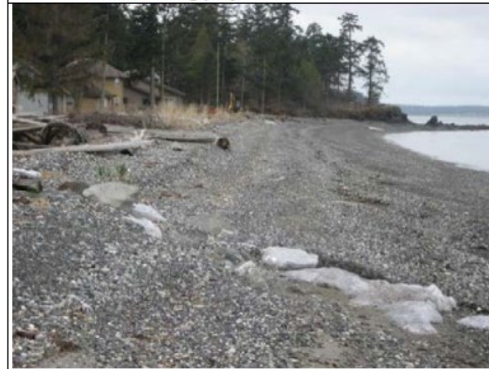
c) North Beach, Orcas Island; western drift sill at end of 510-ft-long project, eastern sill at opposite end (Appendix A).
