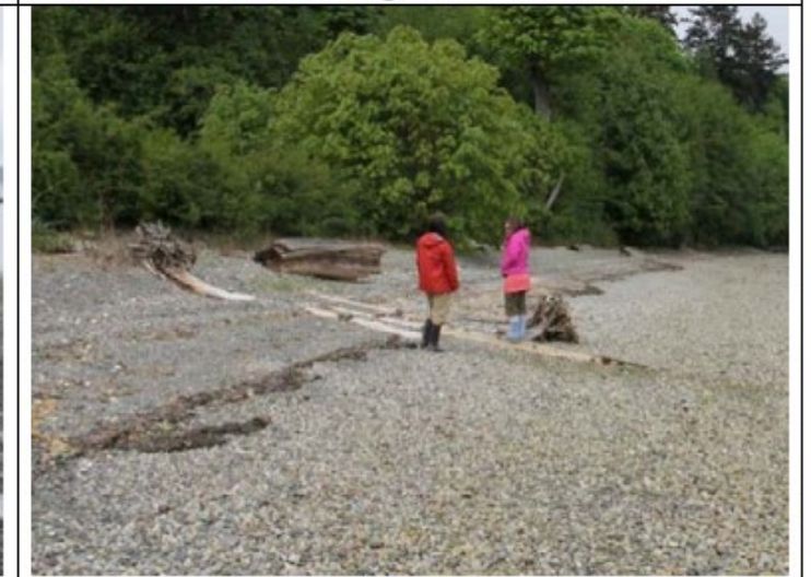
d) Weaverling Spit, Samish Indian Reservation; 1 of 4 large log drift sills within a 500-ft-long project in a highly degraded net shore-drift cell.
