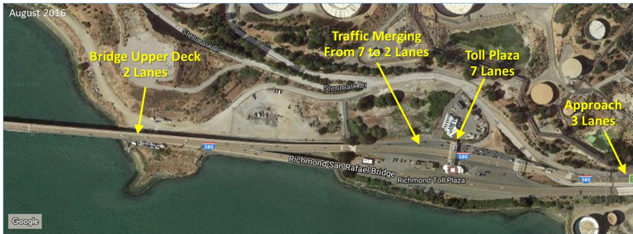
Figure 2-5: Initial Conditions – Westbound Bridge Approach in Richmond
