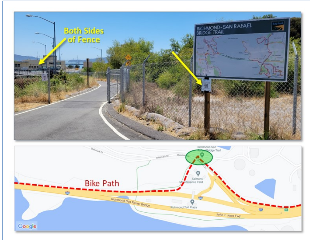
Figure 5-20: User Survey Signs Along Path – Richmond Side
