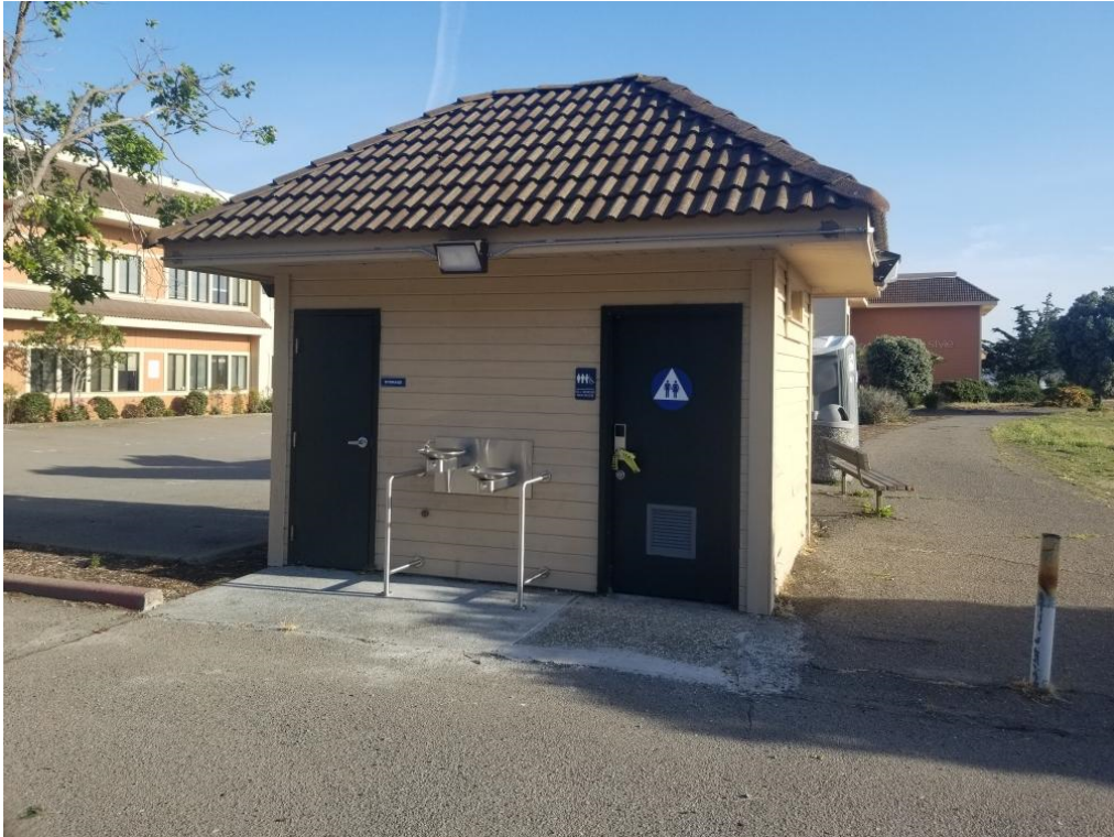
Renovated ADA restroom with exterior lighting and dual level drinking fountain as requested by BCDC. Note ADA accessible temporary bathroom in background.
