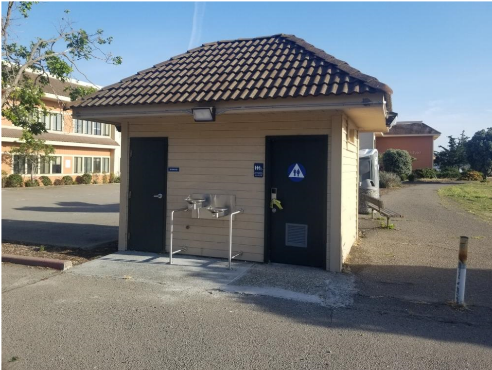
Renovated ADA restroom with exterior lighting and dual level drinking fountain as requested by BCDC. Note ADA accessible temporary bathroom in background.
