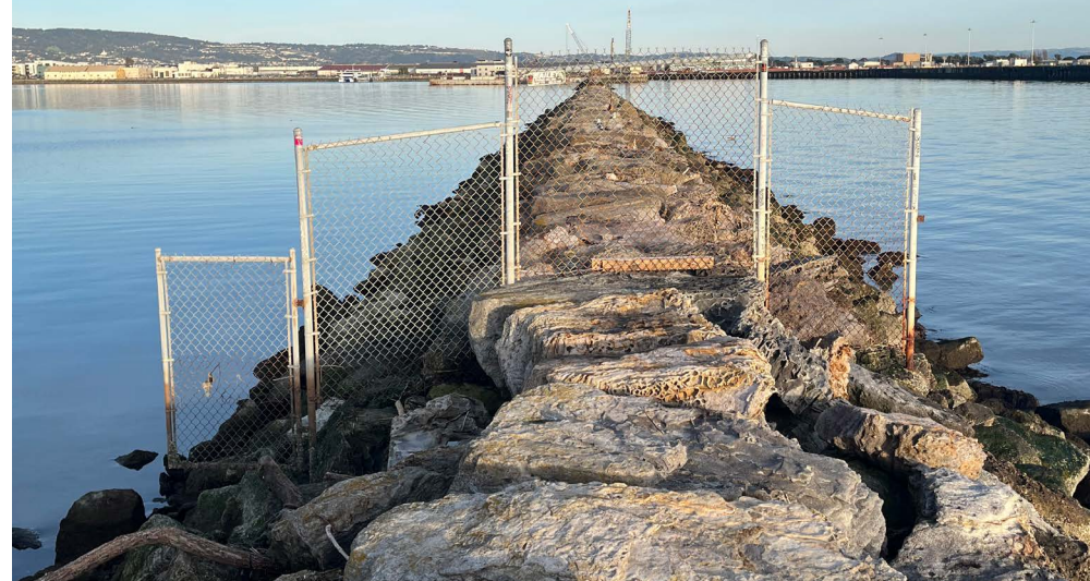
Stone Jetty at the South End of Site
