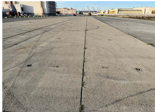
Existing Concrete Re-Use
