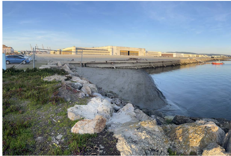
Existing Shoreline at Beach
