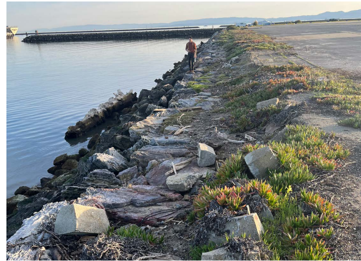
Existing Shoreline Along Axis
