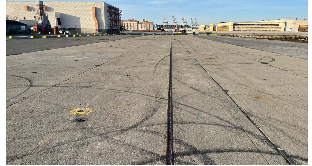
Existing Concrete Paving
