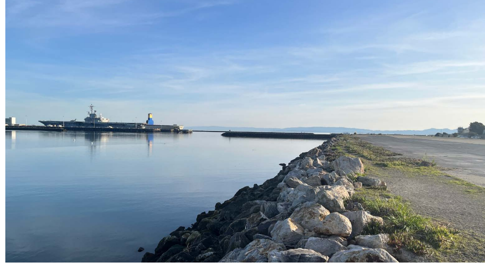
Seaplane Lagoon Armored Shoreline
