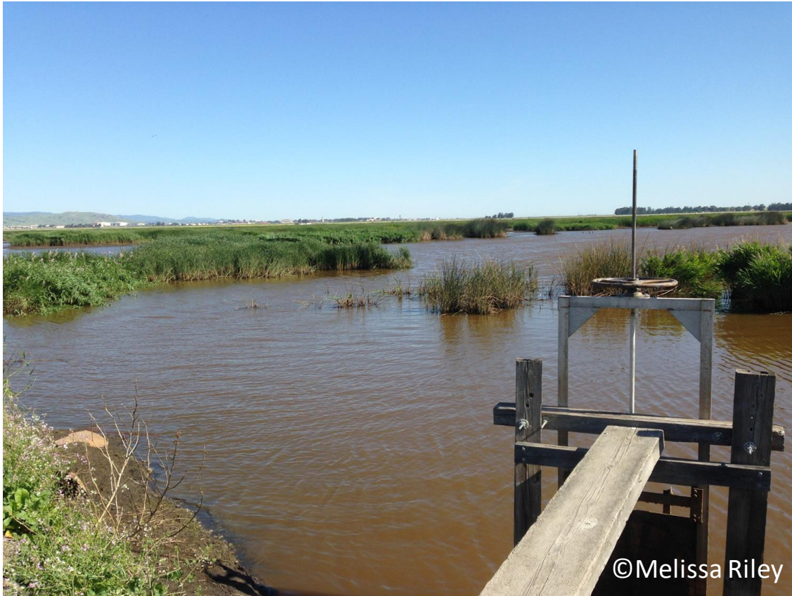
A water control structure being used to flood a managed wetland
