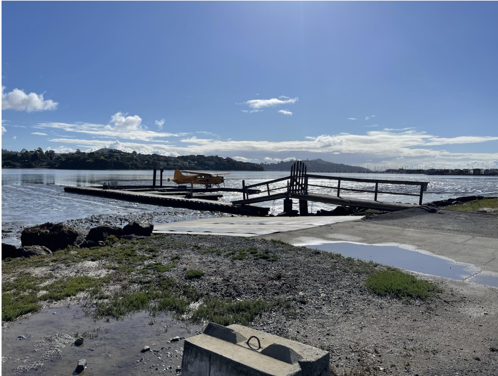
Exhibit 24D. April 22, 2022. Staff photograph depicting completed water access ramp. RED Exhibit C
