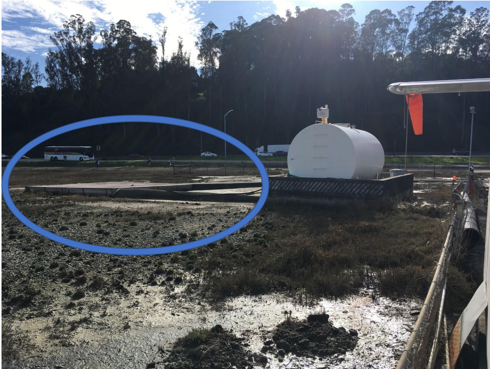
Exhibit 11. January 31, 2020. Staff photograph depicting an unauthorized helicopter landing pad and walkway
