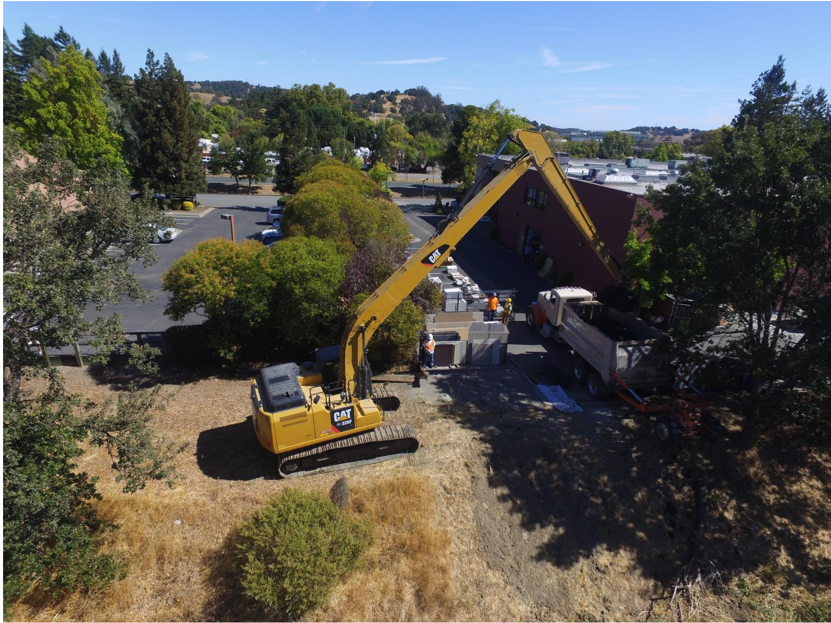
Digging the creek
