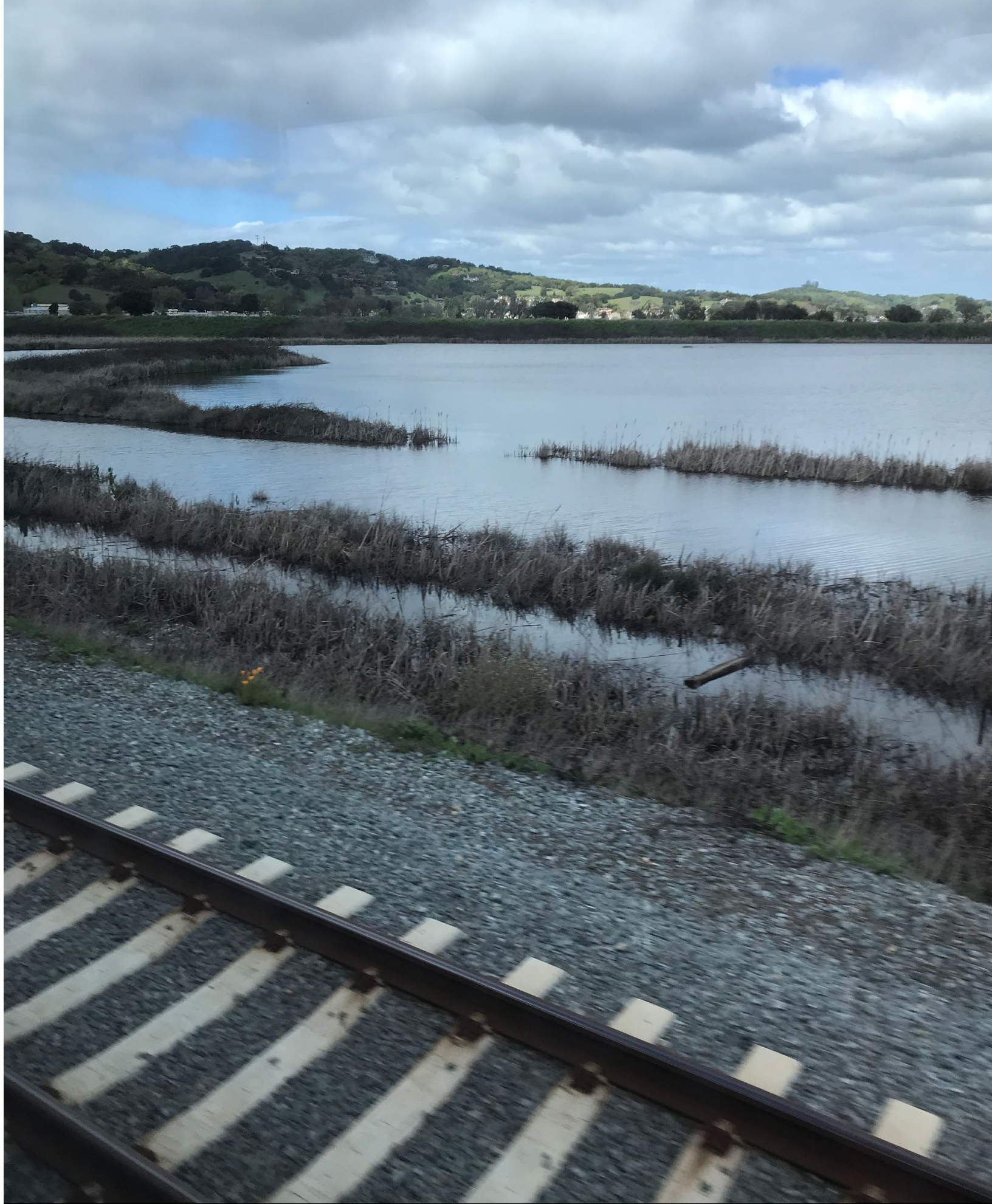
King Tide near SMART rail tracks in Marin. Source: BCDC Staff.
