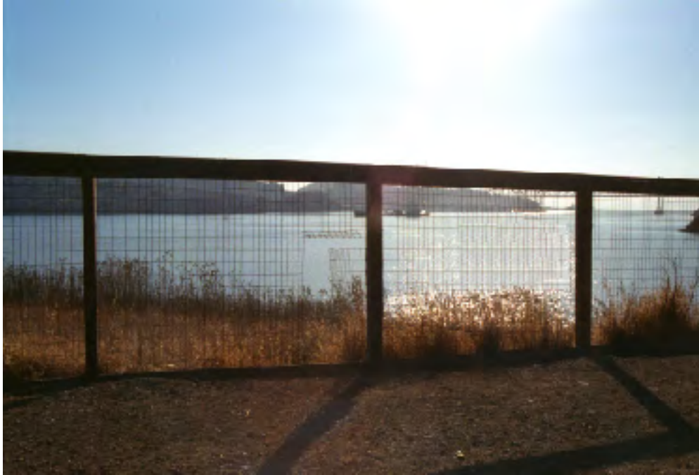
Access not provided to roadway beyond fence, so informal access was created by cutting fence.
