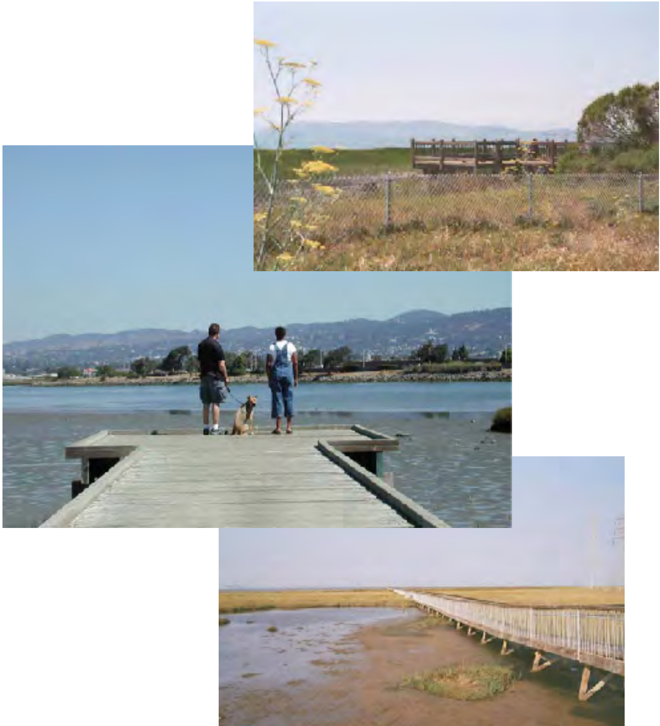
Boardwalks and viewing platforms provide public with physical access to sensitive areas, while confining and structuring human activities.
