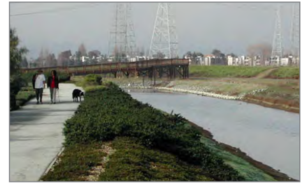
Moats can create a physical barrier while still providing views of the Bay and wildlife areas. Redwood Shores, Redwood City
