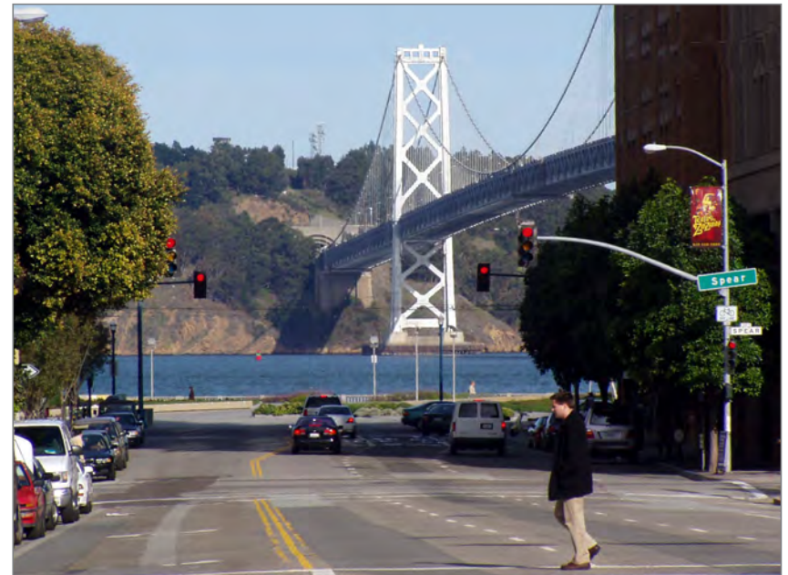
Plan shoreline developments to enhance and dramatize views of the Bay. Folsom Street, San Francisco
