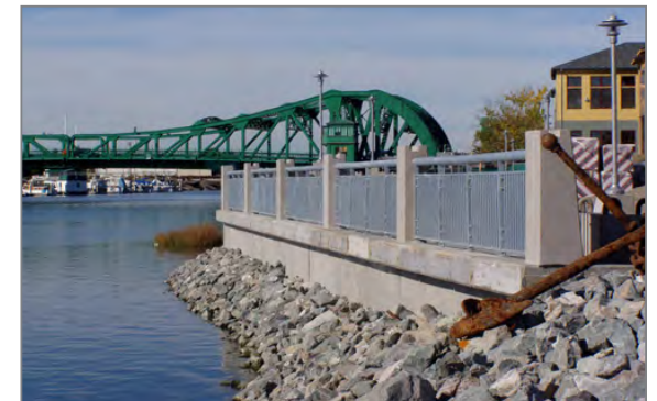
Park Street Bridge, Oakland
