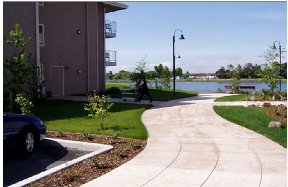
Where development is proposed on long segments of shoreline, public access and views to the Bay should be provided at frequent intervals.
