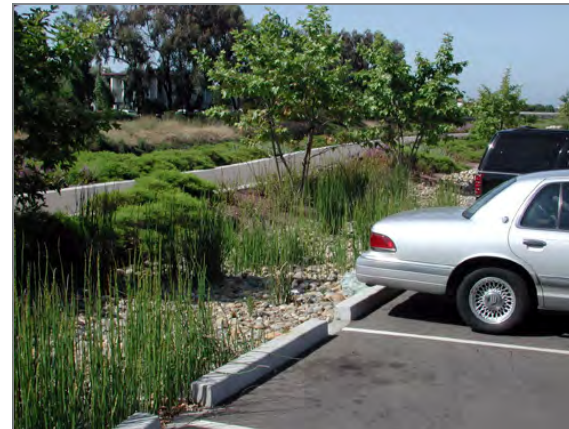
Develop multi-functional stormwater systems. This bioswale screens the parking lot from the shoreline trail. Elmhurst Slough, Oakland
