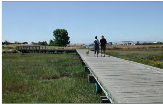
Bridges and boardwalks can confine public use and provide predictability for wildlife while providing physical and visual access. Martin Luther King Regional Shoreline, Oakland
