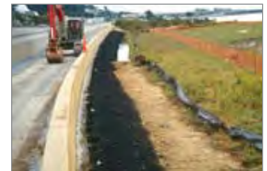
"Honeycomb" mats used for stabilization along Albany shoreline
