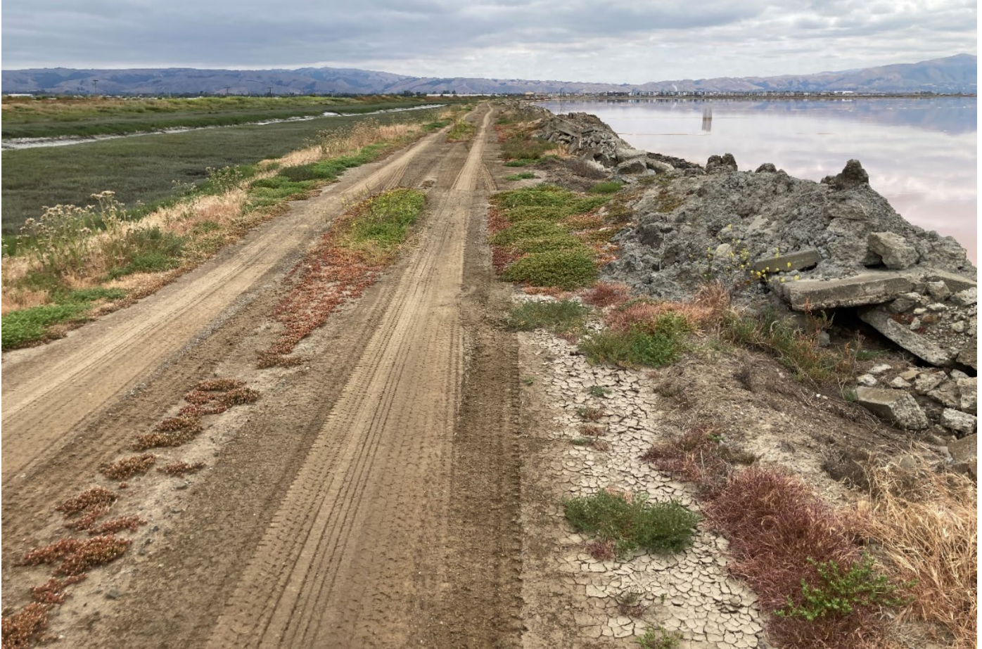
Photo 3. Looking east with the former barge canal on the left and Pond P2-13 on the right. This berm is drivable only during dry weather.
