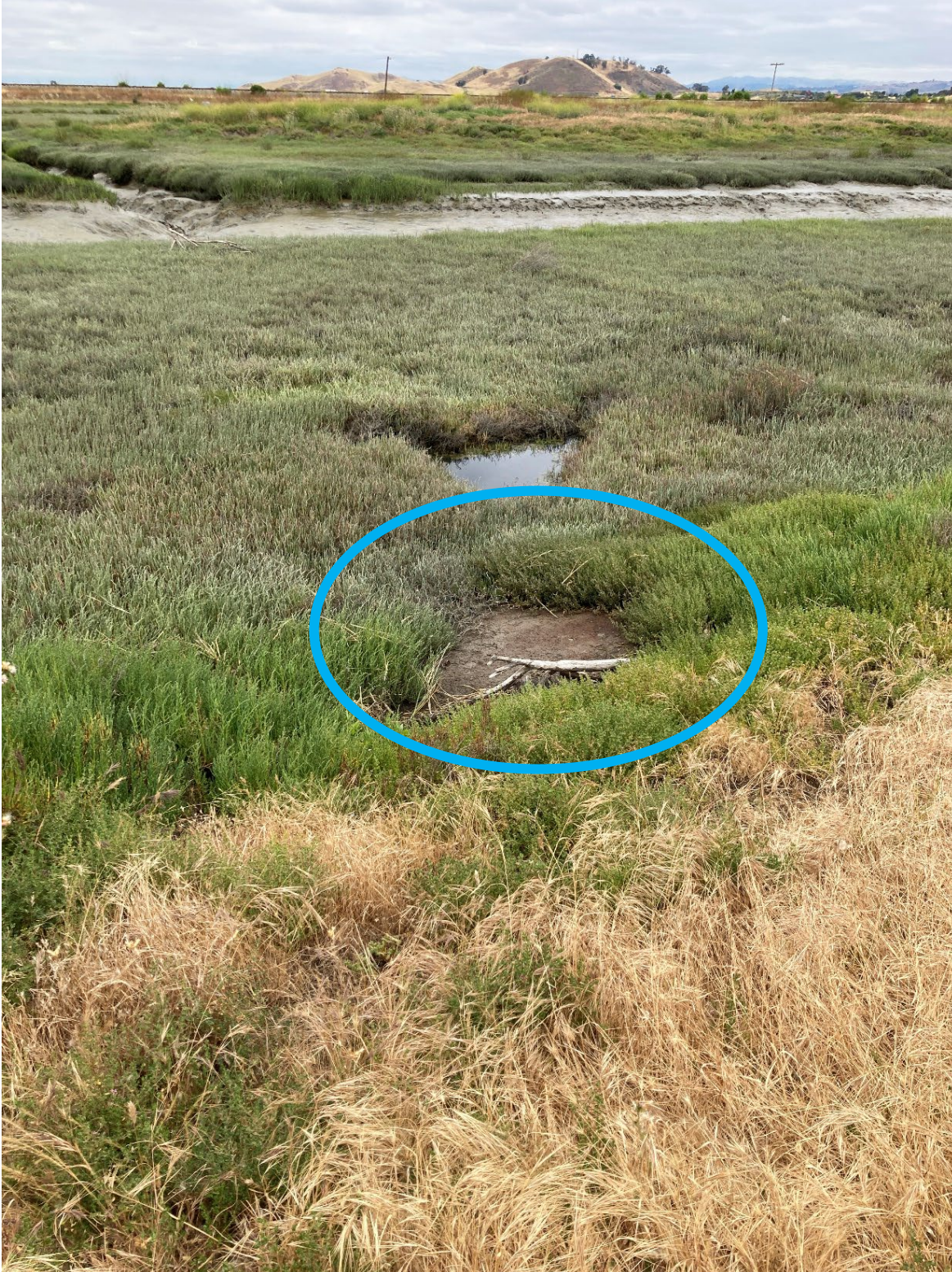
Photo 4. The brown bare spot in the wetland previously showed potential indications of a seep through the berm of Pond P2-13, which Cargill addressed through keying (berm coring).
