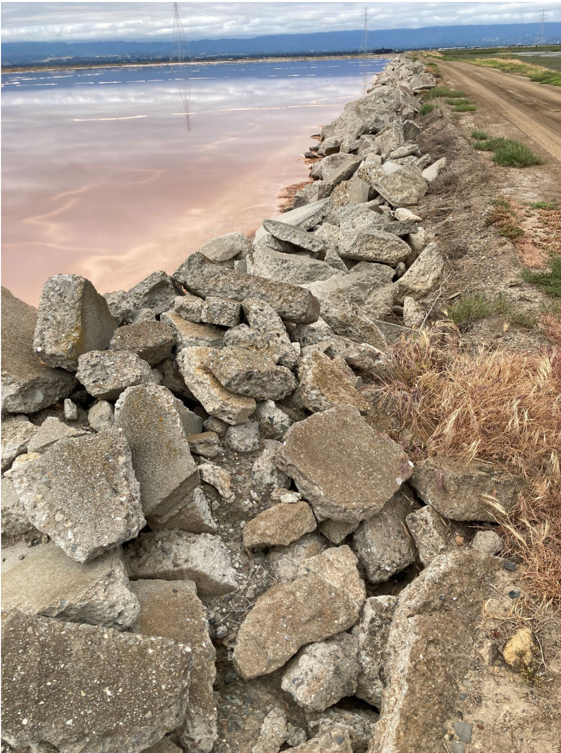
Photo 6. Example of interior berm riprap in Pond P2-13.
