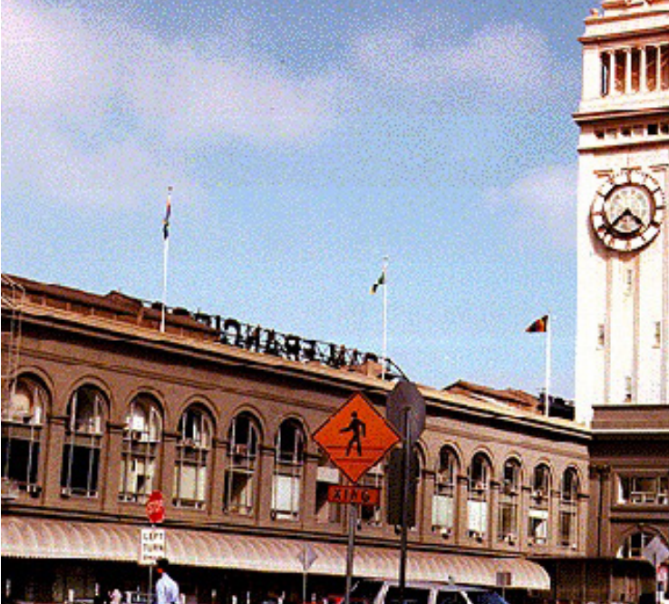
1996, EXTERIOR TREATMENT OF ARCADE
