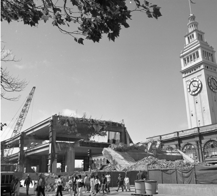
1991, DEMOLITION OF EMBARCADERO FREEWAY
