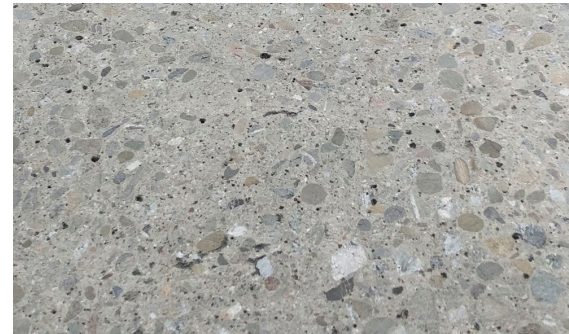
ECOGRIND TREATMENT AT EXISTING PAVING BANDS
