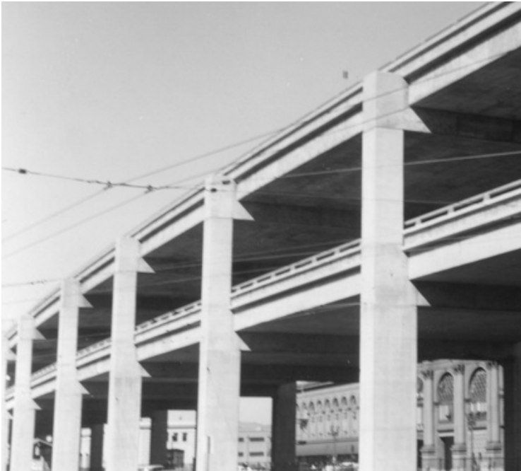
1960, CONSTRUCTION OF EMBARCADERO FREEWAY
