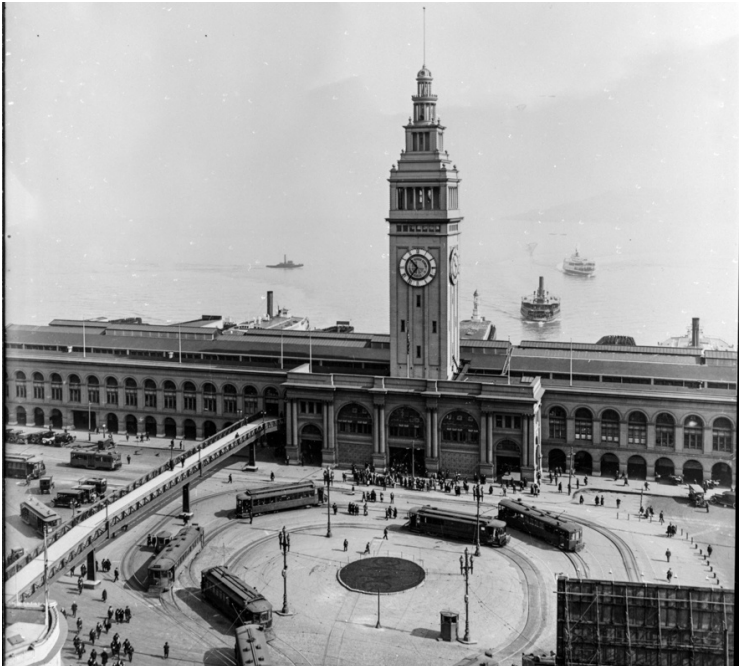
1930, PEDESTRIAN BRIDGE INTRODUCED
