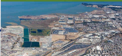
North Richmond Shoreline Living Levee
