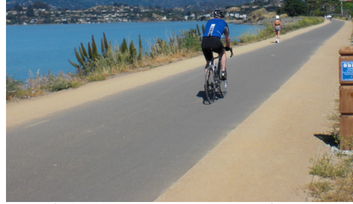
Bay Trail - Asphalt and Crushed Stone Paving
