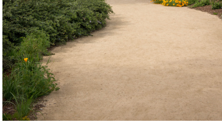
Stabilized Crushed Stone Paving
