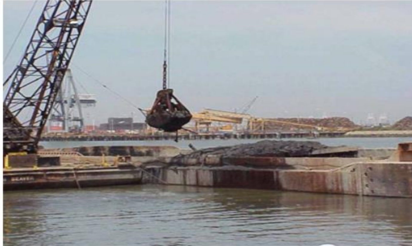
OAKLAND HARBOR DEEPENING – 50 FEET CONSTRUCTION
