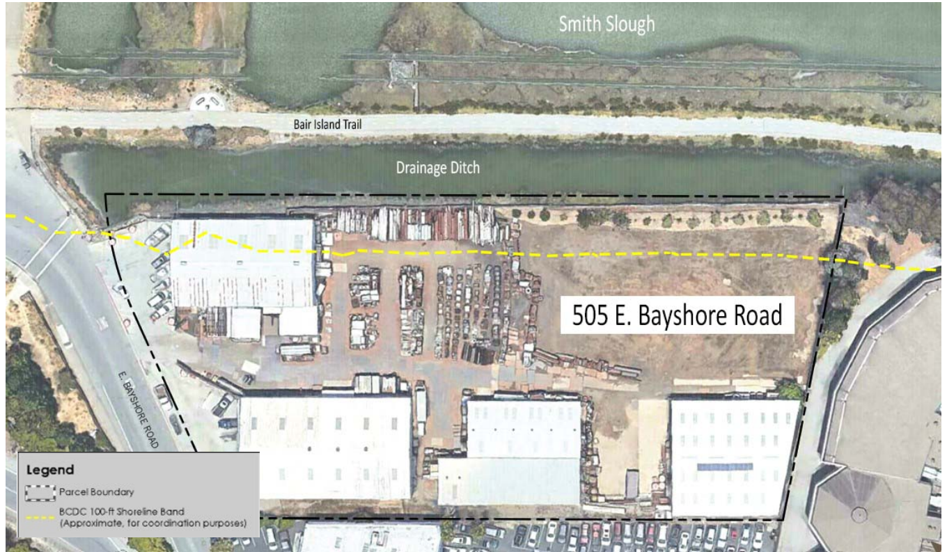
Aerial image of existing site at 505 E. Bayshore Road in Redwood City.
